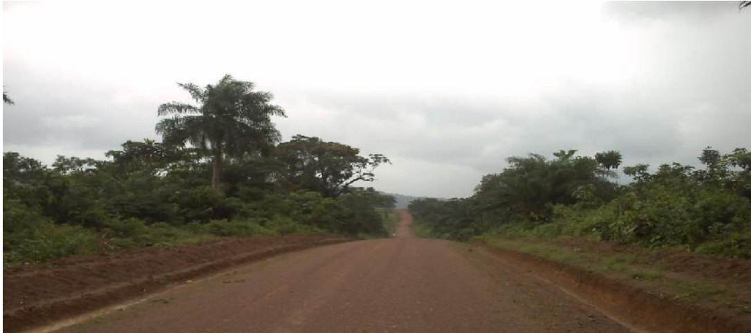
Figure 1 : The newly rehabilitated Nyonbeh Town-Wheasaye (Grand Kola) road .
