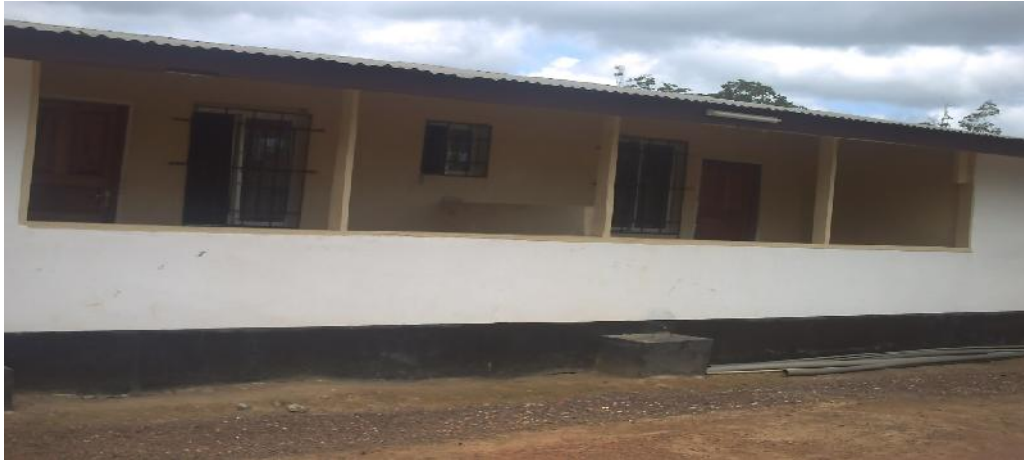
Figure 1: Rented House in Scalepea for the Project Management Team for which US$14,000.00 was paid but not yet occupied after five months
